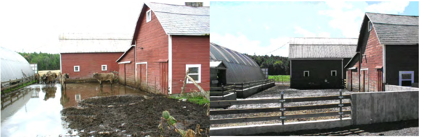
Barnyard before (left) and after (right) surface stabilization using Heavy Use Area Protection (USDA 2014).
