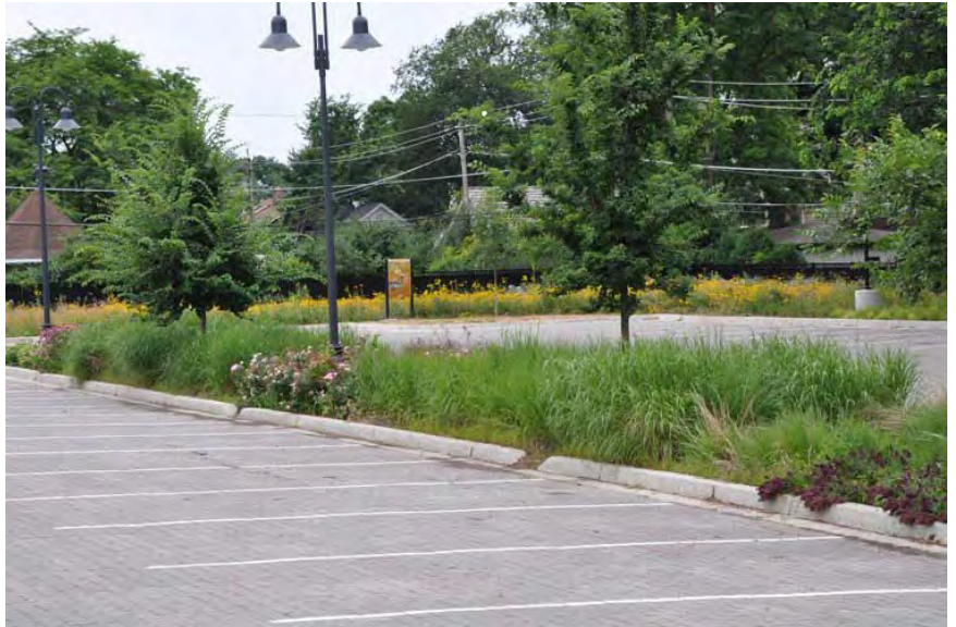
Permeable paving drains into a vegetated swale at Elmhurst College
