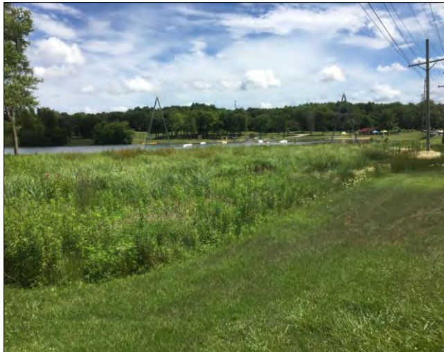
North drainage vegetated Swale
