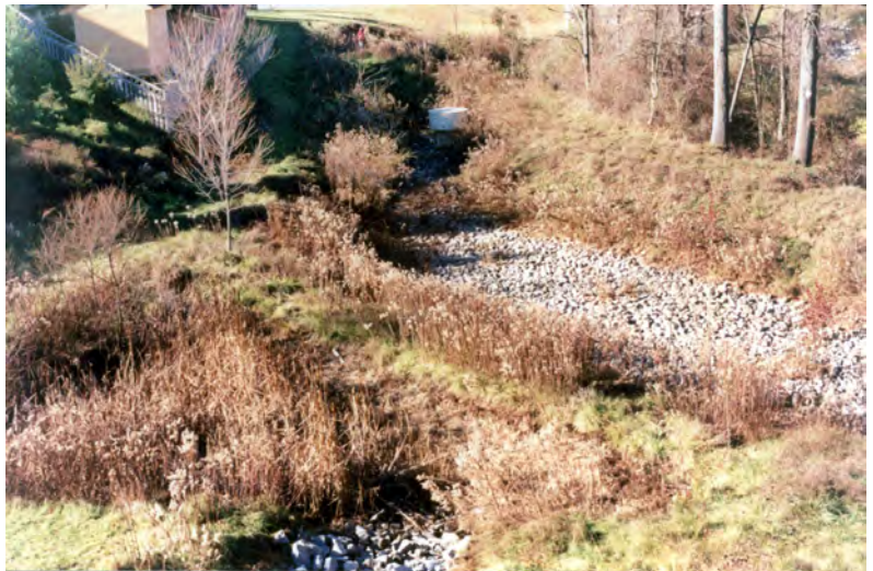
Infiltration trench intermixed with other BMPs (Wikipedia 2018)
