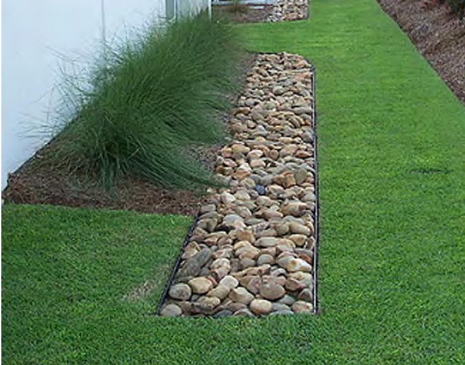
Infiltration trench (Nebraska Stormwater Cooperative 2017)
