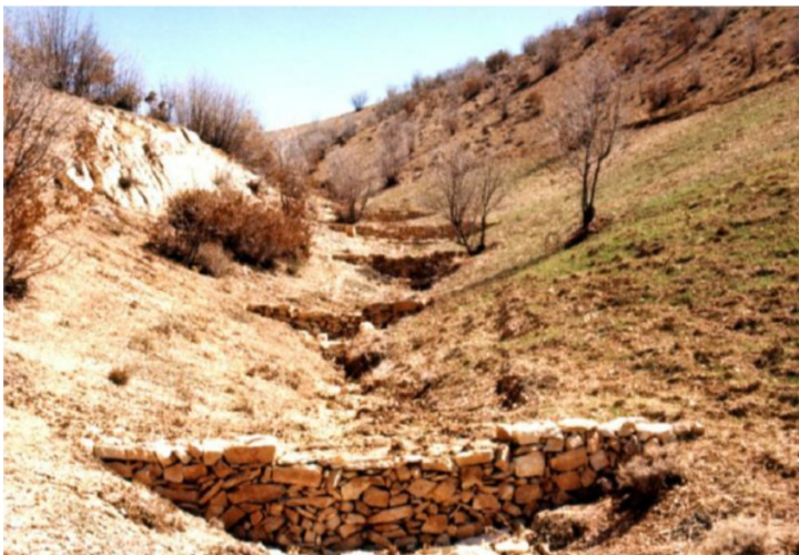
Rock Check Dams ( Source : Hassanli, 2009)
