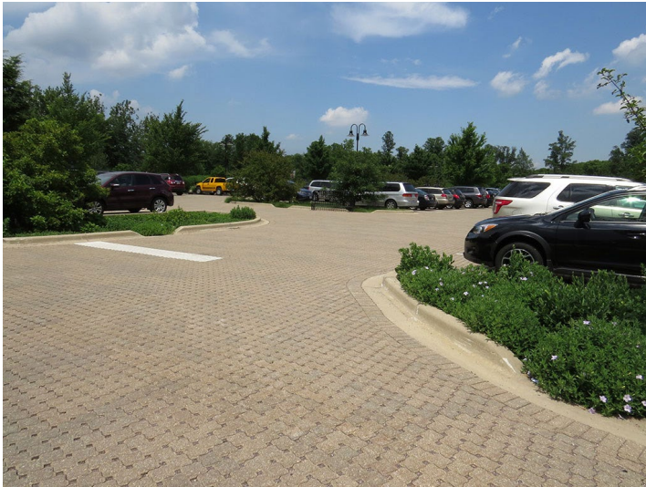
Morton Arboretum, Lisle. Permeable pavers
