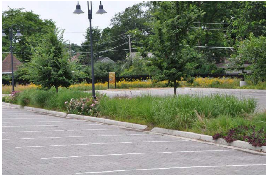
Permeable paving drains into a vegetated swale at Elmhurst College (Jaffe, M., et al 2010)
