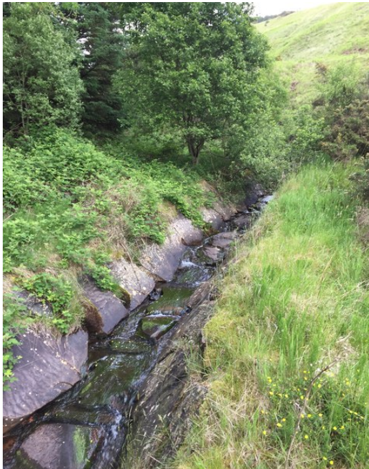
Stone Lined Channel ( Source: Hughes, 2017 )
