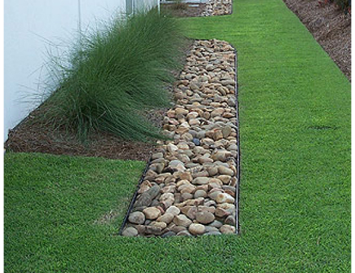
Infiltration trench next to grassed strip ( Source : Nebraska Stormwater Cooperative, 2017)
