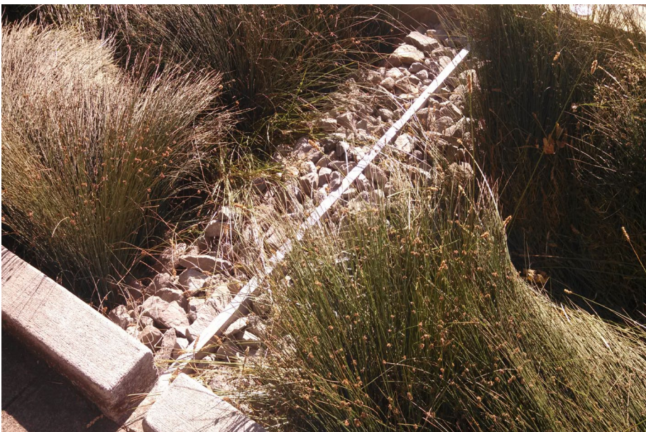
Level Spreader and Vegetative Strip (Source: Kirk)
