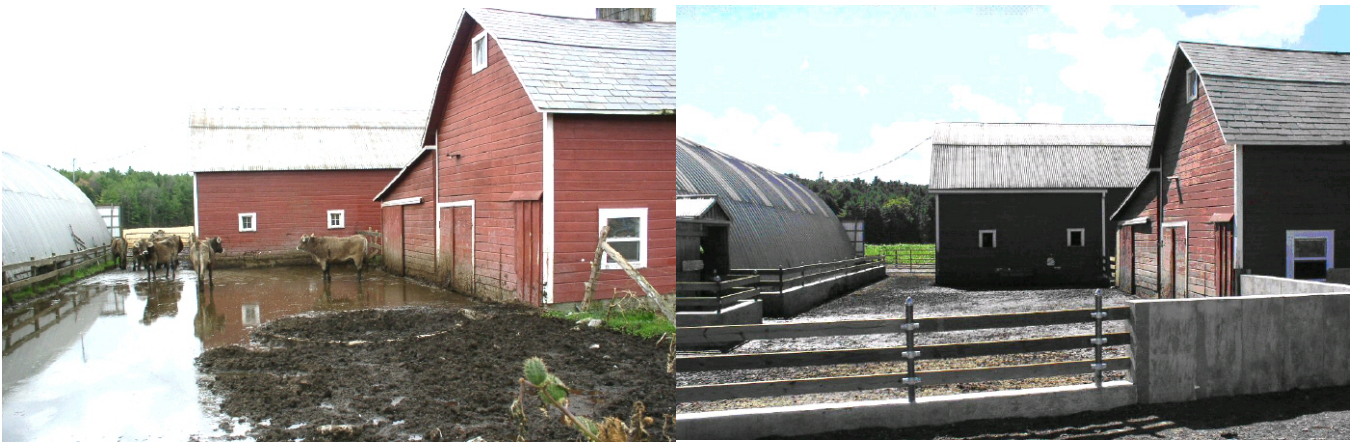
Barnyard before (left) and after (right) surface stabilization using Heavy Use Area Protection ( Source : USDA, 2014).
