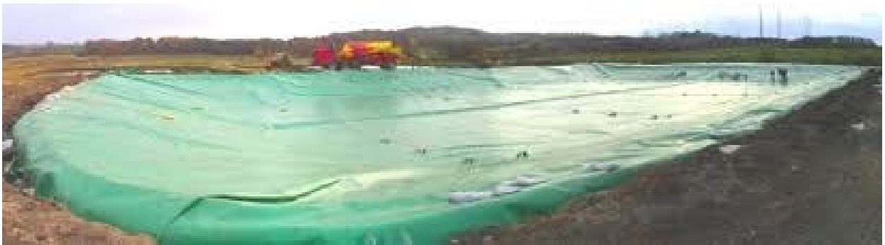
Cover over an agro-waste management facility (Source: NRCS, 2015)
