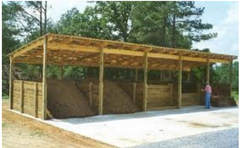
Slanted wooden roof over compost facility (Source: NRCS, 2015)
